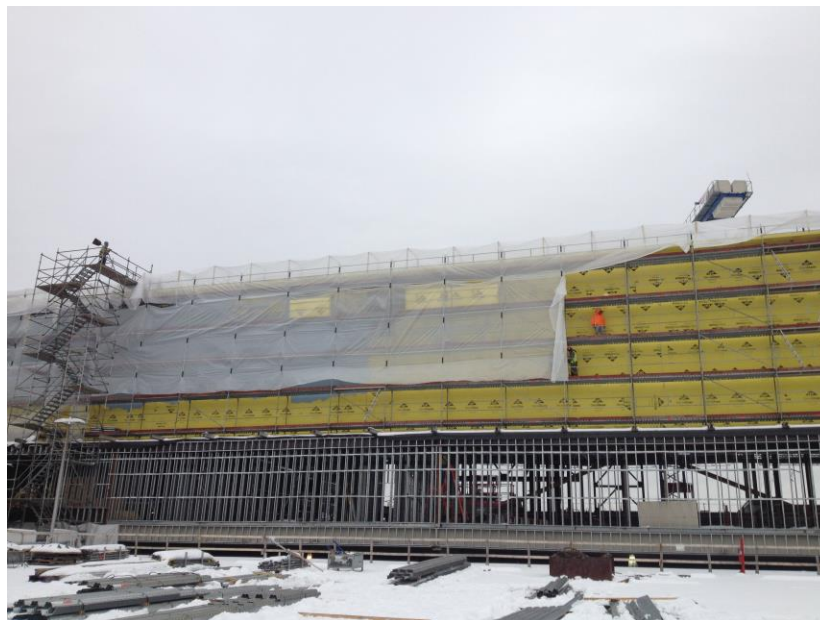
Figure 3.4 – Original Exterior Envelope Installation
