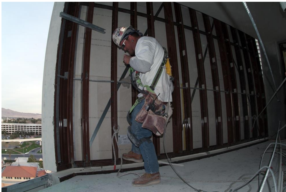
Figure 3.5 – KHS&S Prefabricated Wall Installation
